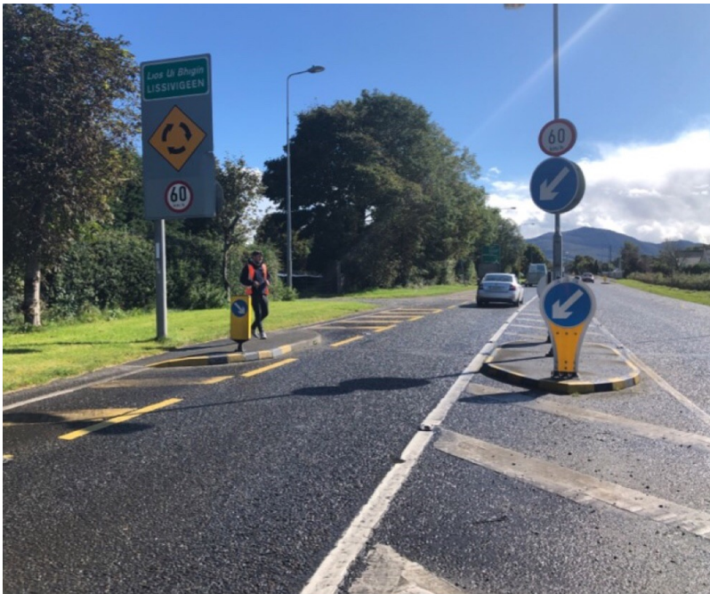
Location 38 - N22 Splitter Island At Entry To Lissivigeen Direction Continue On N22 Visual inspection indicates that loaded blade component will navigate with no issues. *Note* Road width - 3.8 Sign to sign - 5.8
